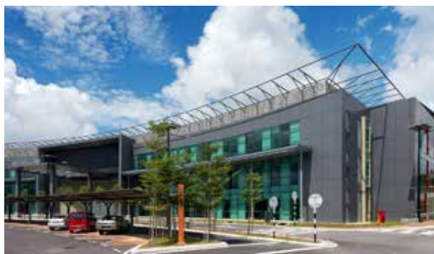
Medical Rehabilitation Block
