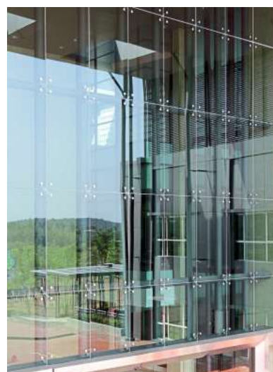
The low-emissivity glass panels reflect away 60-70% of the heat hitting the building, helping to keep the insides cool and cooling costs low.
