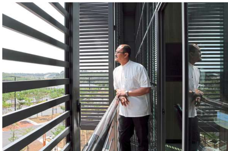
Mokhlis on a balcony outside one of the offices showing the louvred screens that can be opened to let in more air and light.
