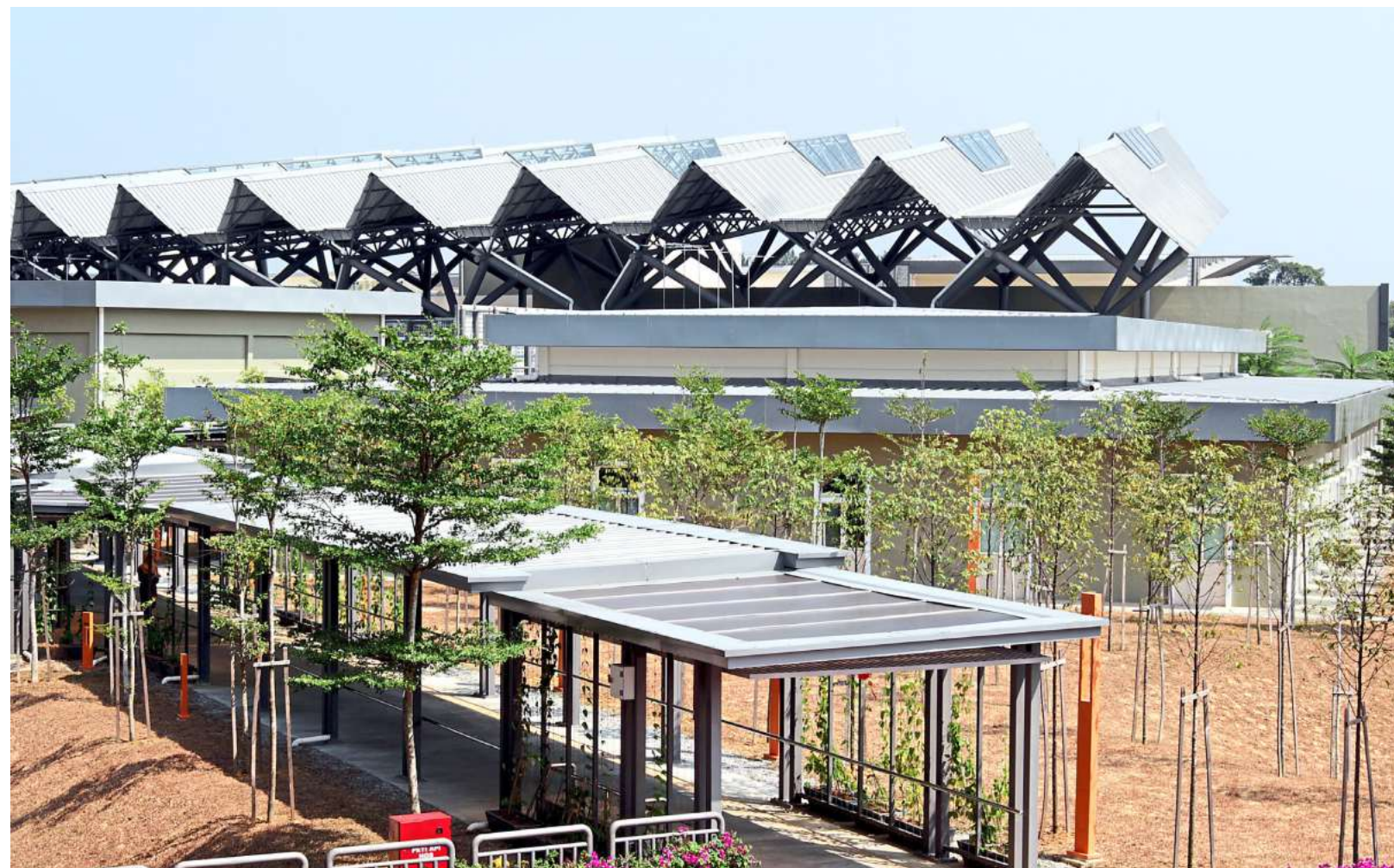
Naturally cool: The folding fan-inspired steel roof over the Sanctuary Garden at the Socso Rehabilitation Centre in Malacca acts as a wind tunnel and promotes air flow. Photos: SAM THAM/The Star
