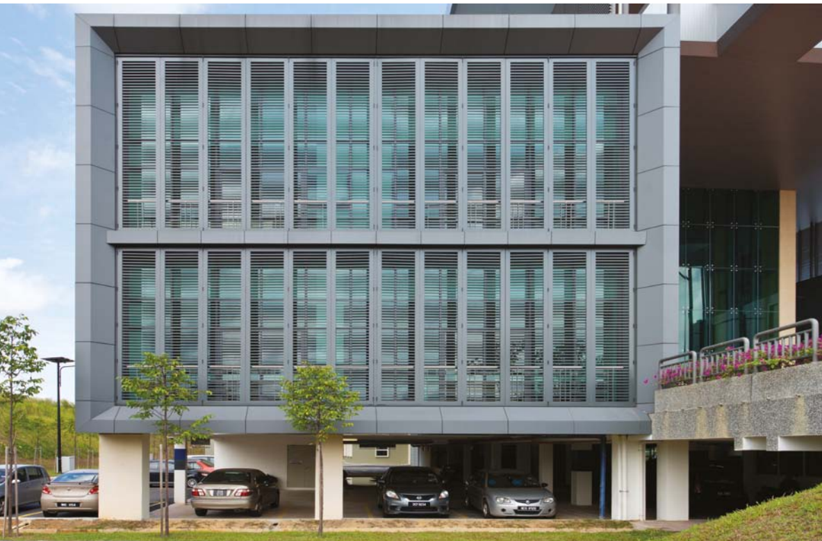
ABOVE: Admin Block main facade with sun shading open; BELOW: Admin Block main facade with sun shading closed
